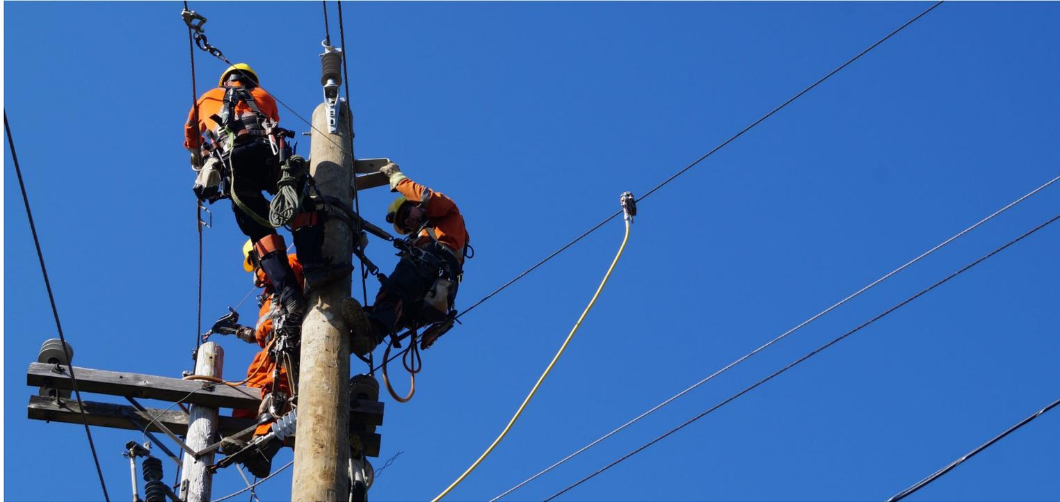
Photo: Crews replacing a crossarm structure.
