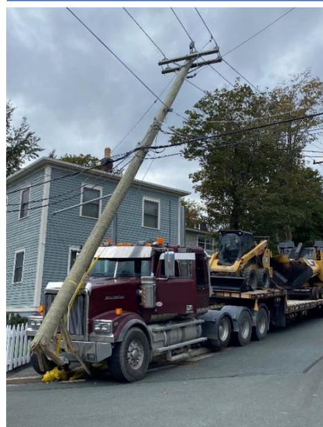
One public contact incident in the quarter involved heavy equipment damage to a pole in St. John’s. A customer outage was required to make repairs.
